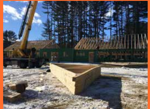
Construction as of February 14.
